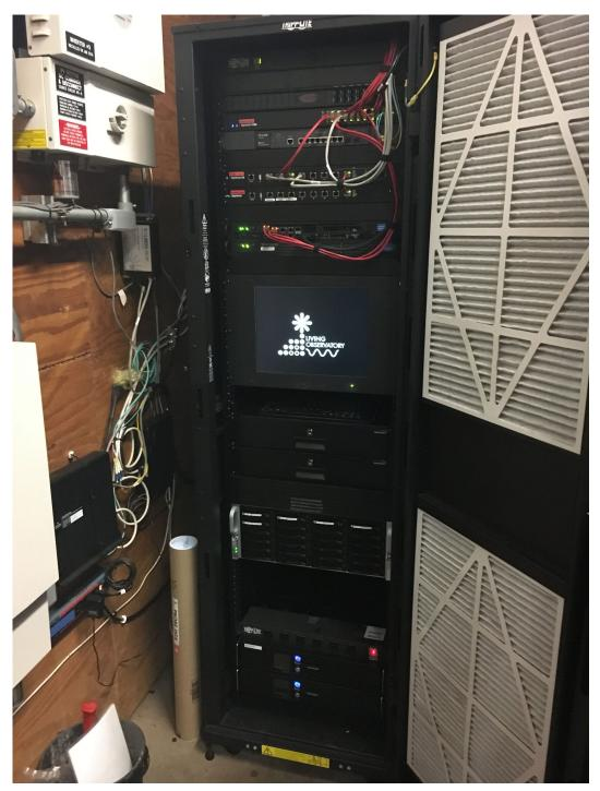
Figure 3.8: The indoor portion of the Tidmarsh network head end.
