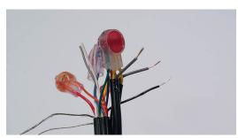
(m) Step 13. Strip the Ground Wires
